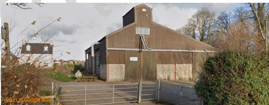
Figure 19 Typical agricultural building situated within the area north of the A43
