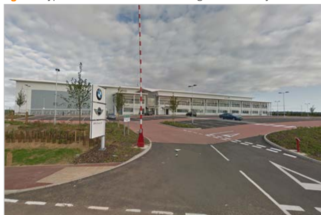
Figure 6 Typical distribution Centre building in Swan Valley
